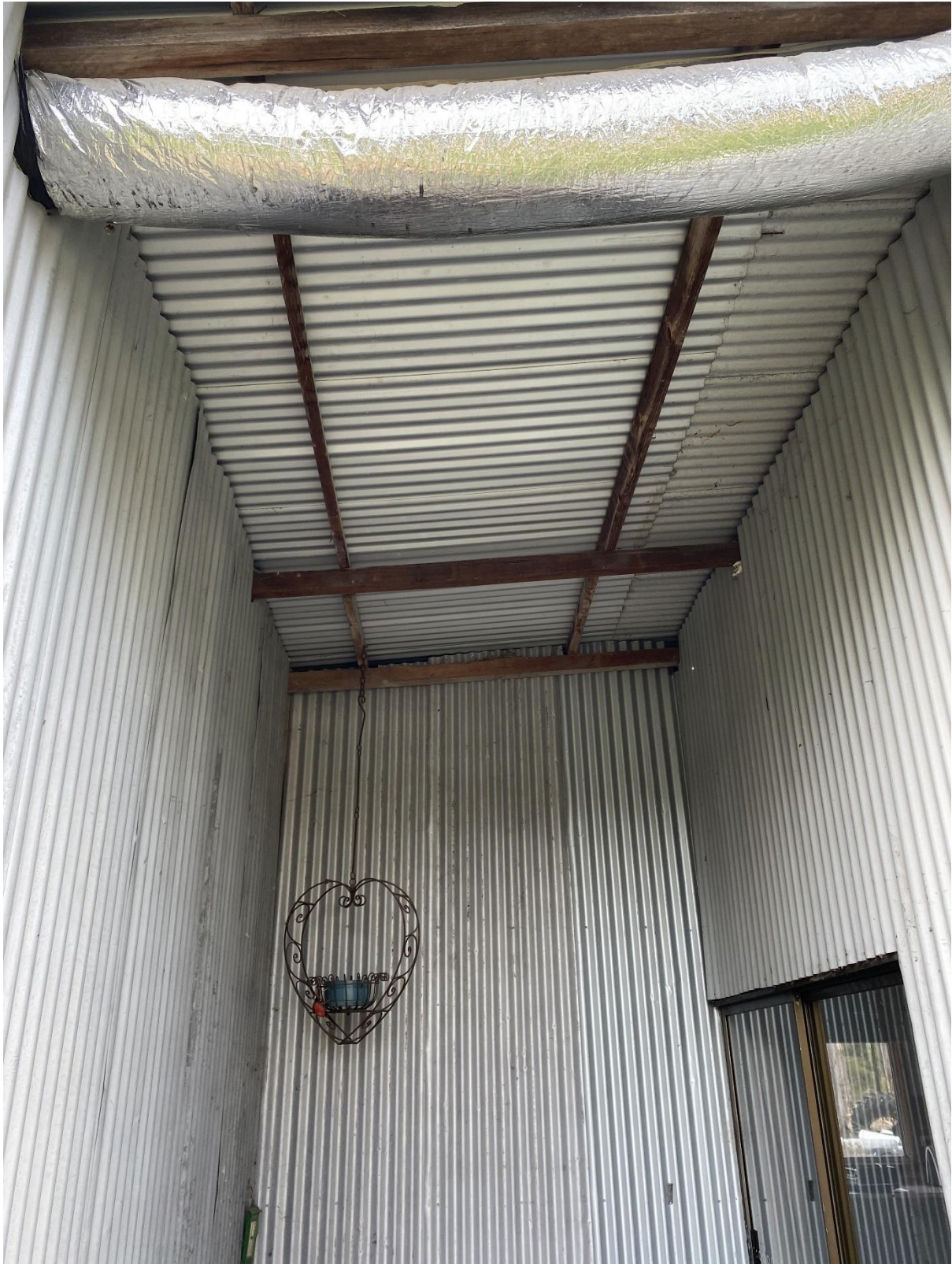
Photograph 6 – Shed structure entry roof. Rafters spacing too large.
