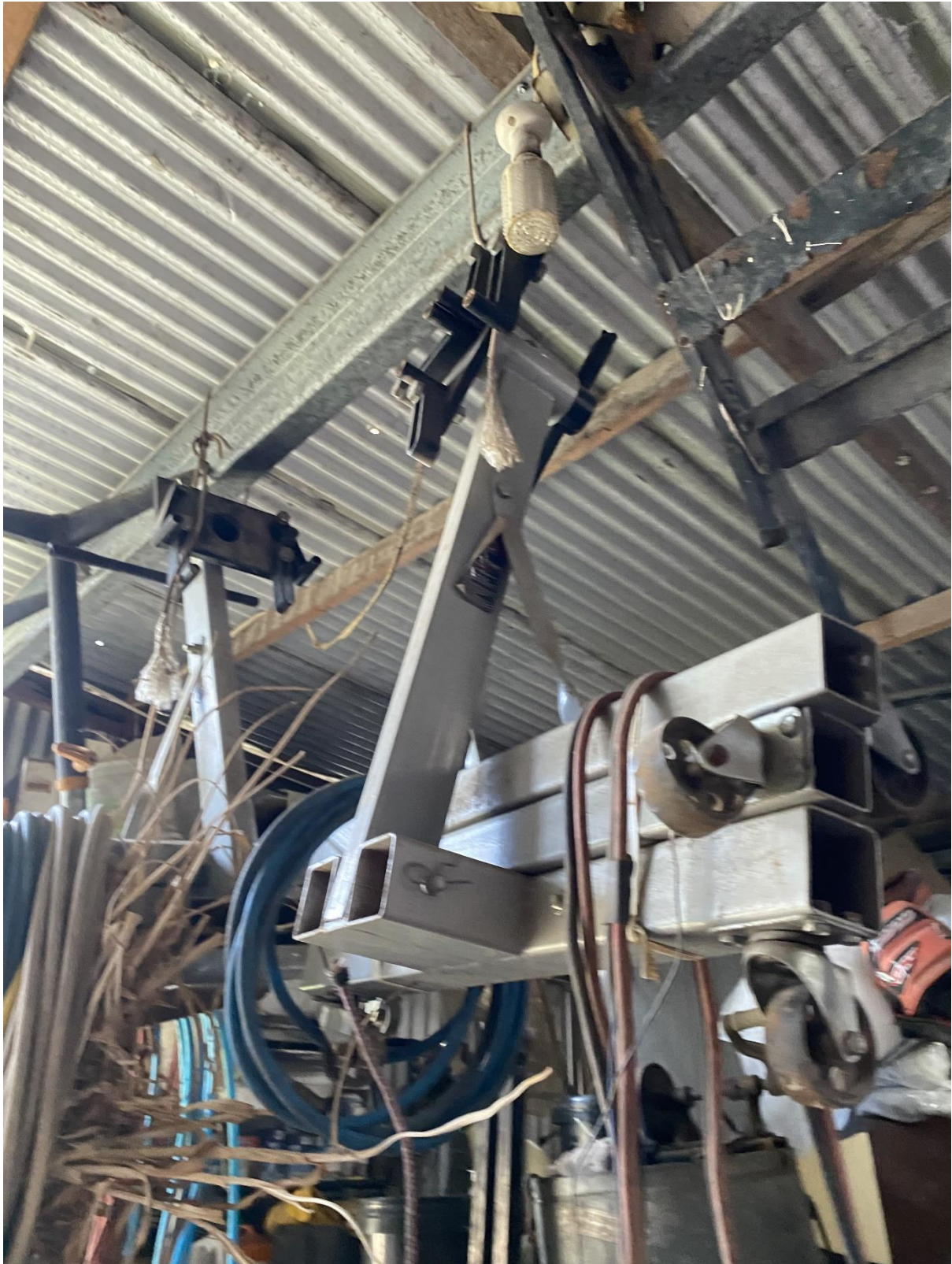
Photograph 7 – C200 purlin beam requires two additional post supports to reduce span.
