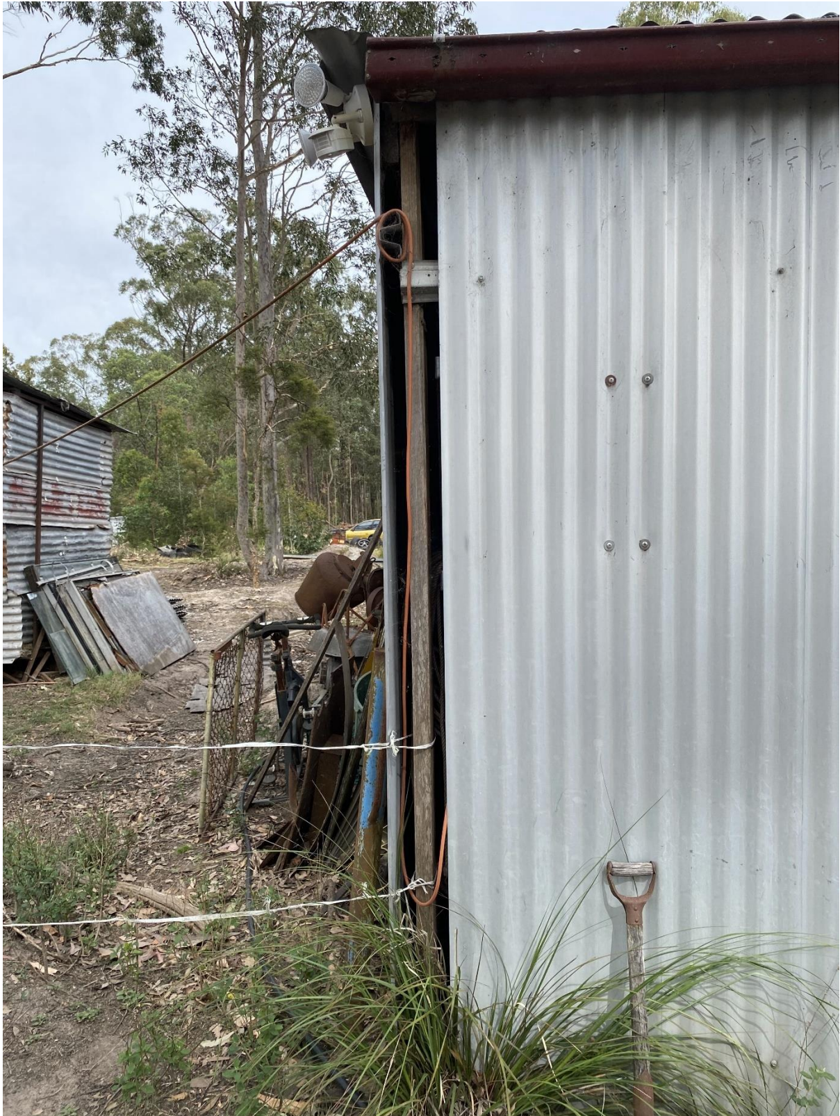
Photograph 9 – Shed structure wall batten spacing too large and fixings missing.
