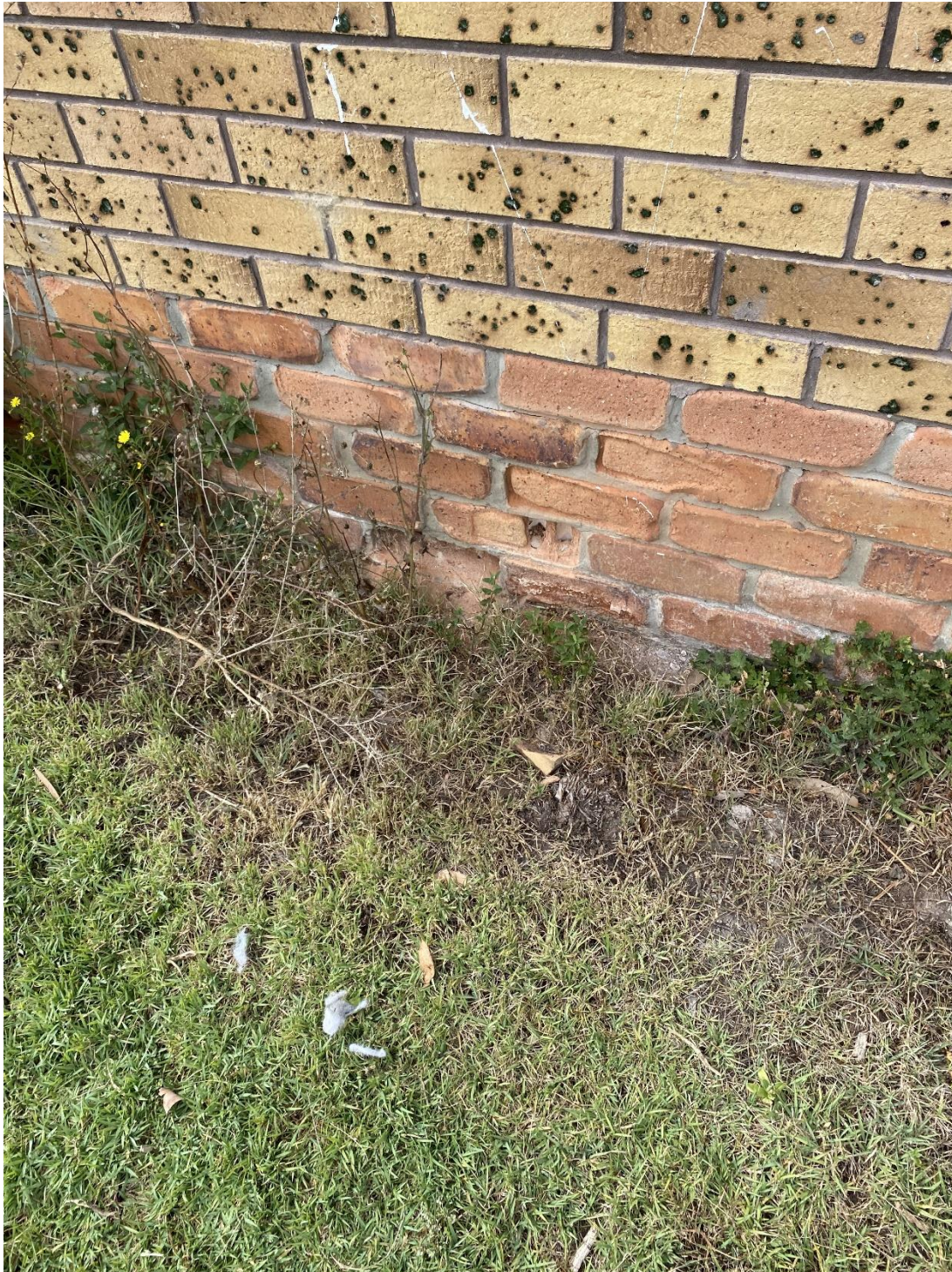
Photograph 3 – Deterioration of subfloor masonry on single storey dwelling.
