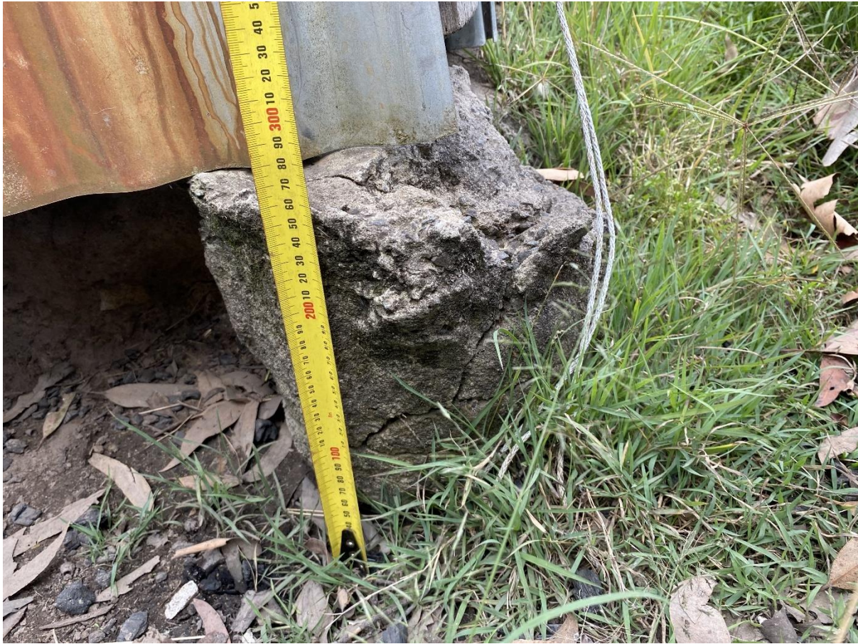
Photograph 10 – Shed structure pad footing undermined and undersized.
