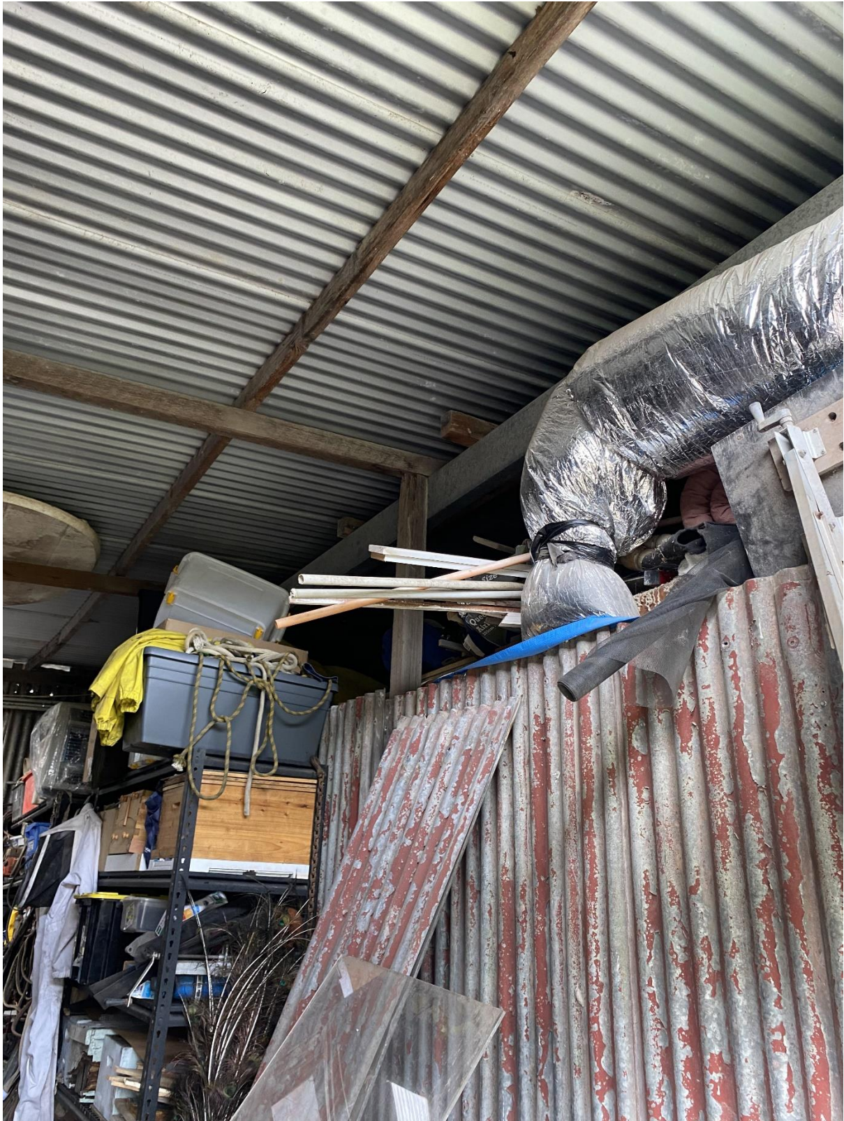
Photograph 8 – Shed rafter spacing too large. Add rafters to reduce spacing.
